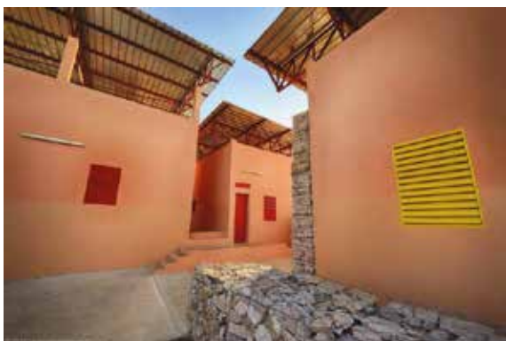
ORPHELINAT FALATOW JIGIYASO _ F8 ARCHITECTURE, DIALAKOROKA, MALI
