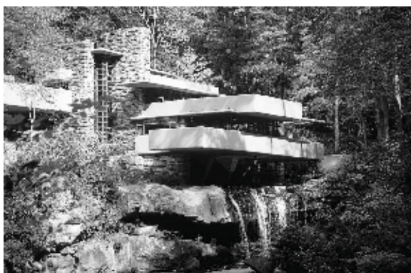
FALLINGWATER HOUSE _ FRANCK LLOYD WRIGHT, ETATS-UNIS, (1935)
