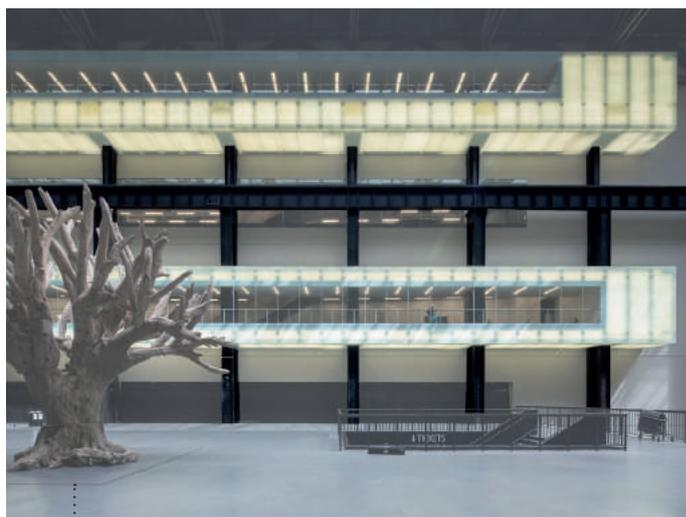
BOÎTES D'ACIER INSÉRÉES DANS LA STRUCTURE EXISTANTE
